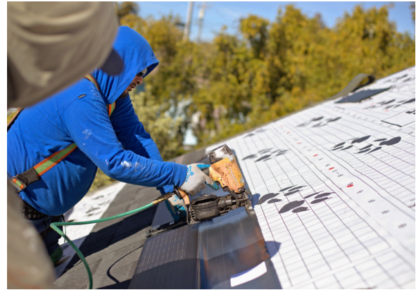
Energy shingles being installed
