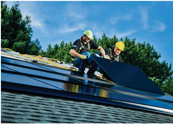
Solar panels being installed
